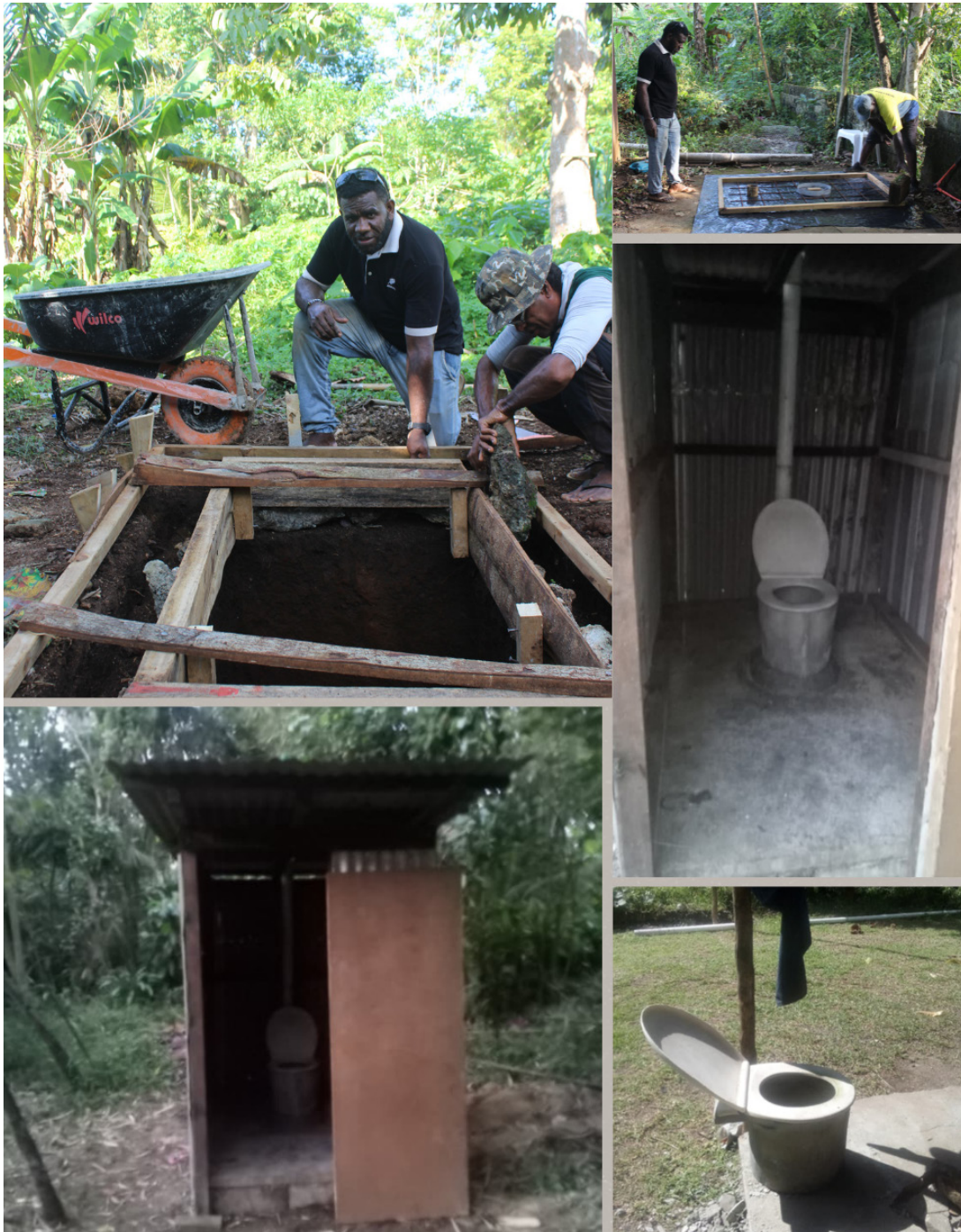
(After the WASH training William, he has become a champion in supporting community to construct safe VIP for community HH.)
